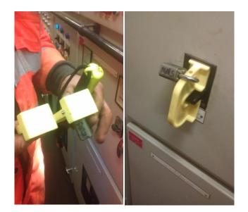
Failure of the lockout equipment used to isolate switch consoles in the engine control room of a marine aggregate dredger resulted in a Near Miss during a recent maintenance stop at a ship yard.
